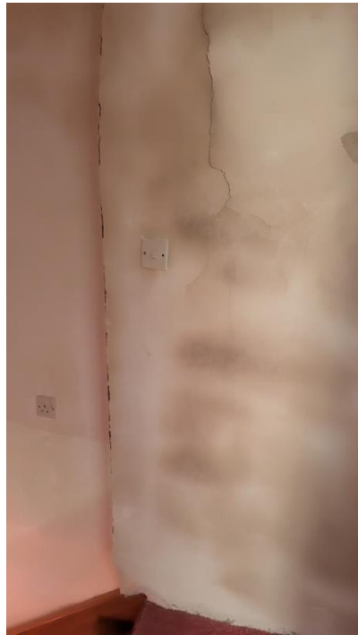
Above: widespread damp and mould issues in the two modern extensions.
