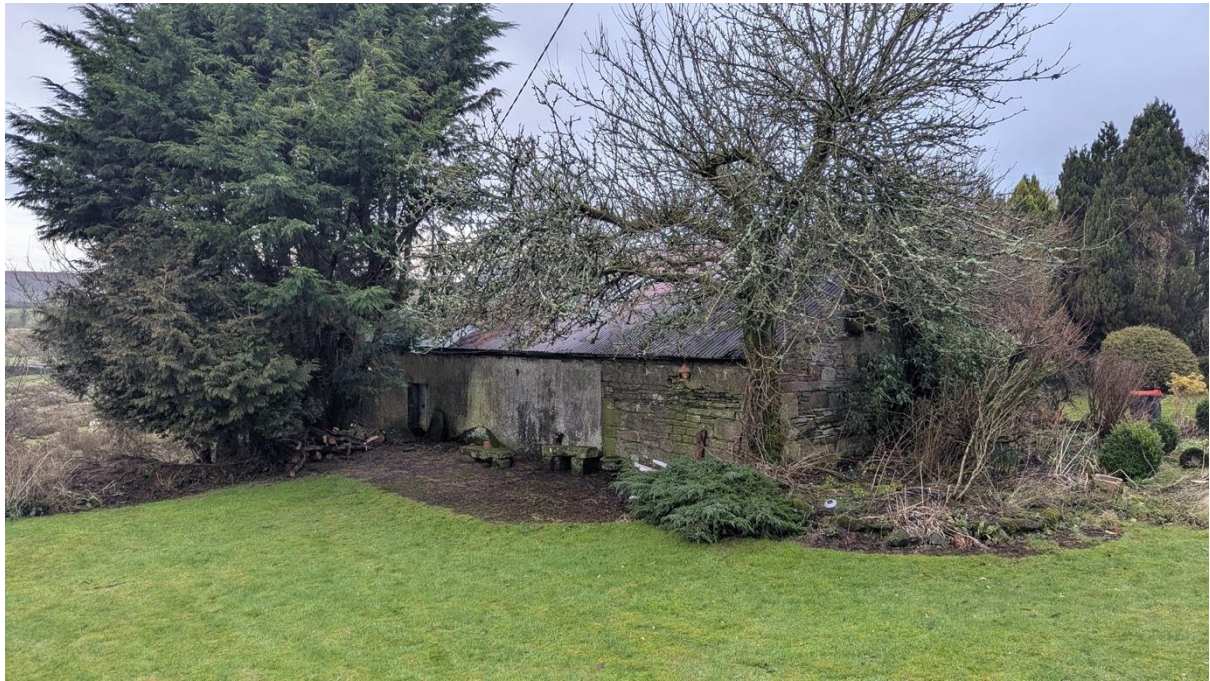
Above: photo facing north west towards the southern elevation of the byre, as taken from the garden area. The byre is partly obscured by trees from this viewpoint. Sections of render and exposed stone can be clearly seen on this elevation. An unused well is situated behind the byre which has been covered over.
