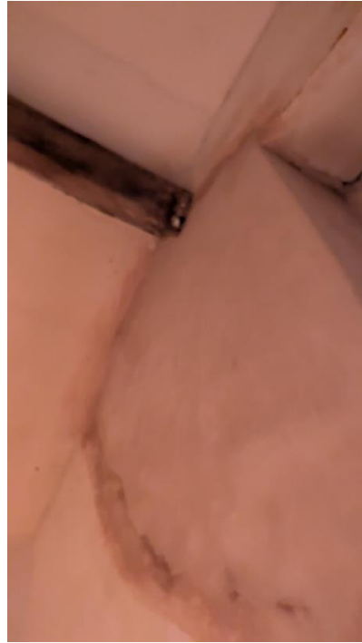
Above: widespread damp and mould issues in the two modern extensions.
