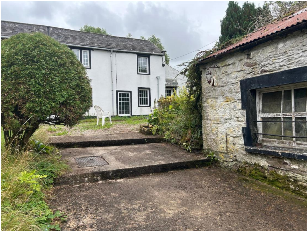
Above: photo showing the relationship between the eastern end of the byre and the main house. The stone of the byre has been limewashed at some stage, and the stone surrounds painted black. Concrete steps split the level difference between the byre and driveway and the main house. Here, the modern extensions to the house can be defined by the drainpipe on the front elevation and include the ground floor multi-pane glazed door, single to ground and first floor and the mono-pitch lean-to extension.
