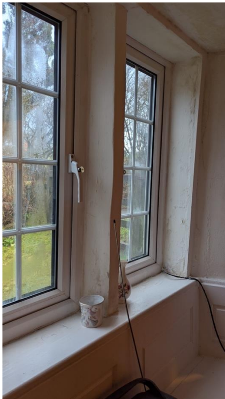
Above L: modern plaster and paints have been applied to the internal stone mullions of the windows in the original house. This along with internal warmth has caused damp issues as seen here. It is proposed to remove these modern products allowing the stone to breathe, lime will be used in its place. It is proposed to remove the UPVC window units and replace them with slim double glaze timber/metal alternatives as shown on the plans accompanying this document. Above R: photo showing the southern elevation of the lean-to extension. The oil tank is accessed from this side of the building.
