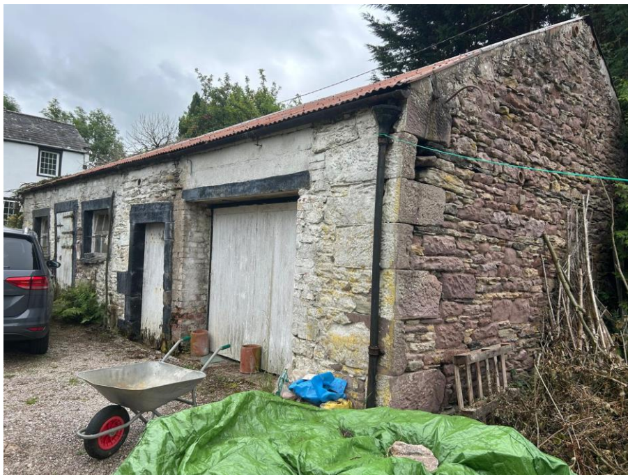
Above: photo facing the northern elevation and western gable of the byre. Here the dressed sandstone can be clearly seen. Also, sections of limewash and concrete block infill sections where door alterations have been made over time. It is proposed to clean and repoint the stone work and removal harmful products such as anything cementitious or paint.
